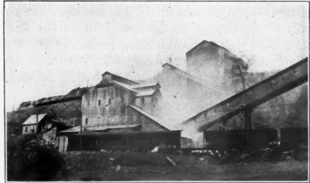
Crushing Plant, with Conveyor Housing at Right
